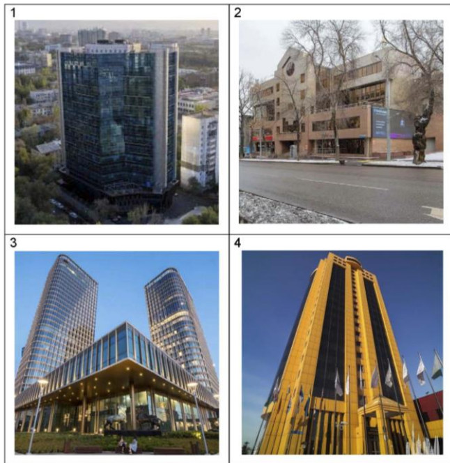
Figure 1. Certified business centers in Kazakhstan: 1 – the «Park View Office Tower», Almaty; 2 – the «Prime Business Park», Almaty; 3 – the «Talan Towers», Astana; 4 – the «Astana Tower», Astana
