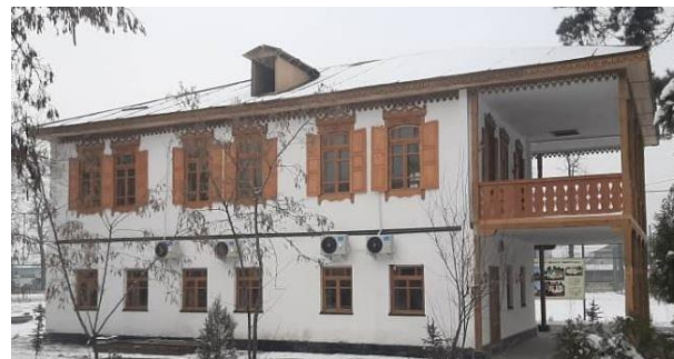
Figure 5. The house of the mayor of Pishpek I. Terentyev. Restoration in 2023
