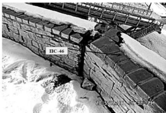
Figure 1. Defective retaining wall design
